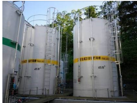
NaClO storage tanks
