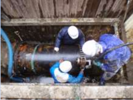
DIP-K \phi 800 repairing
