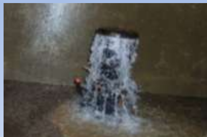
Air valve damage
