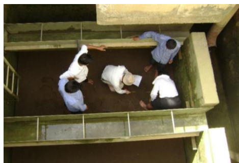
Inspection of filter sand layer OJT in phase 2 (Battambang water treatment plant)
