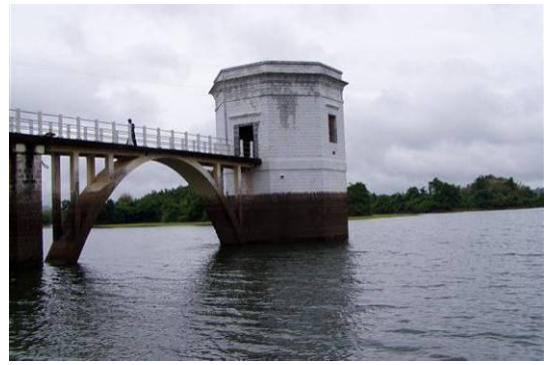
Intake tower in reservoir, Yangon
