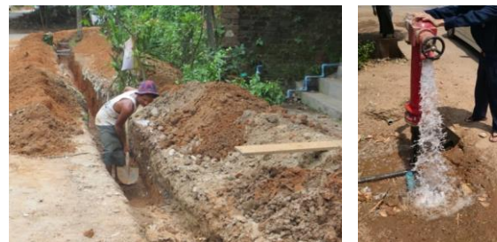
Figure 7 Digging for laying pipes & water supply after completion of the project
