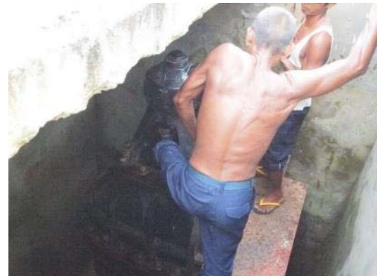
At a valve near a pumping station. It takes 45 minutes to open/close a valve manually.
