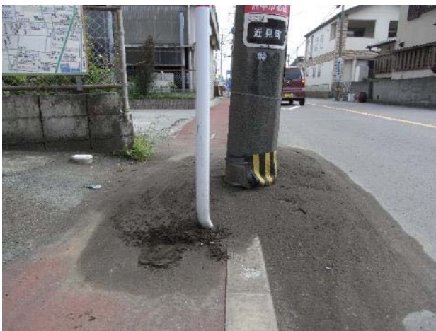
Situation of liquefaction in eastern Kumamoto City. The sign on the utility pole shows displacement depth.
