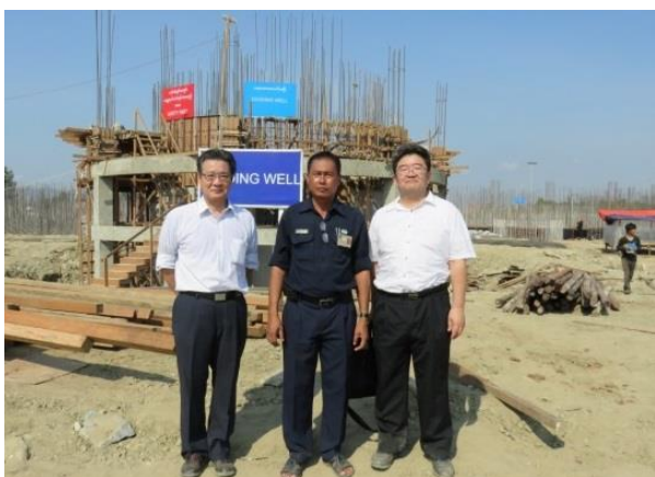
At construction site of new WTP (from left: Mr. Kinugasa, Mr. Zaw Min, Nagashio)
