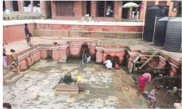
The use situation (pattern) of public tap ✘ In the case of a large-scale facility, water supply by natural water is not enough, and it is used after being stored in a tank once
