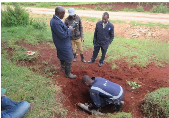
Verification of passing flow rate using UFM
