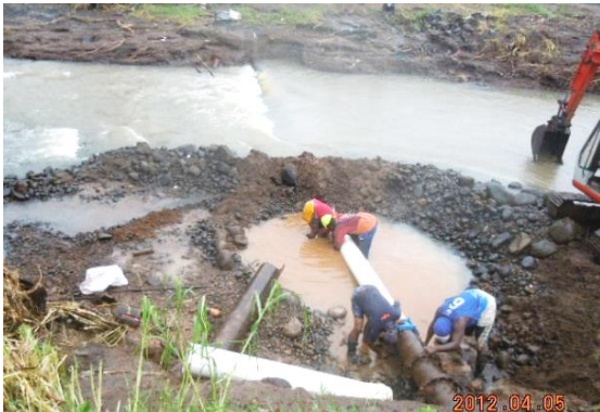
Photo 4: Piping work (repairing leakage) in water
