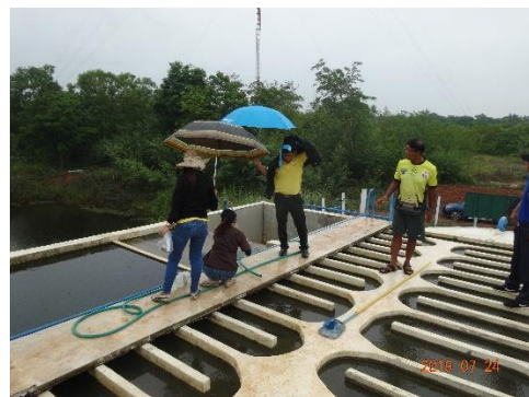
Fig. 2 Actual water purification plant
