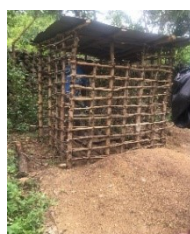
Latrine built by residents
