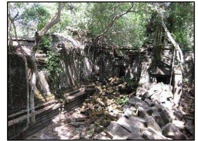
Photo: Collapsing ruins
