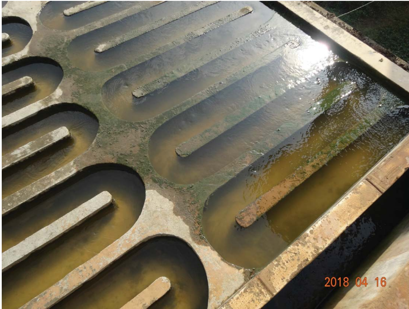
flocculation basin with no flow, overflow, and algae attachment
