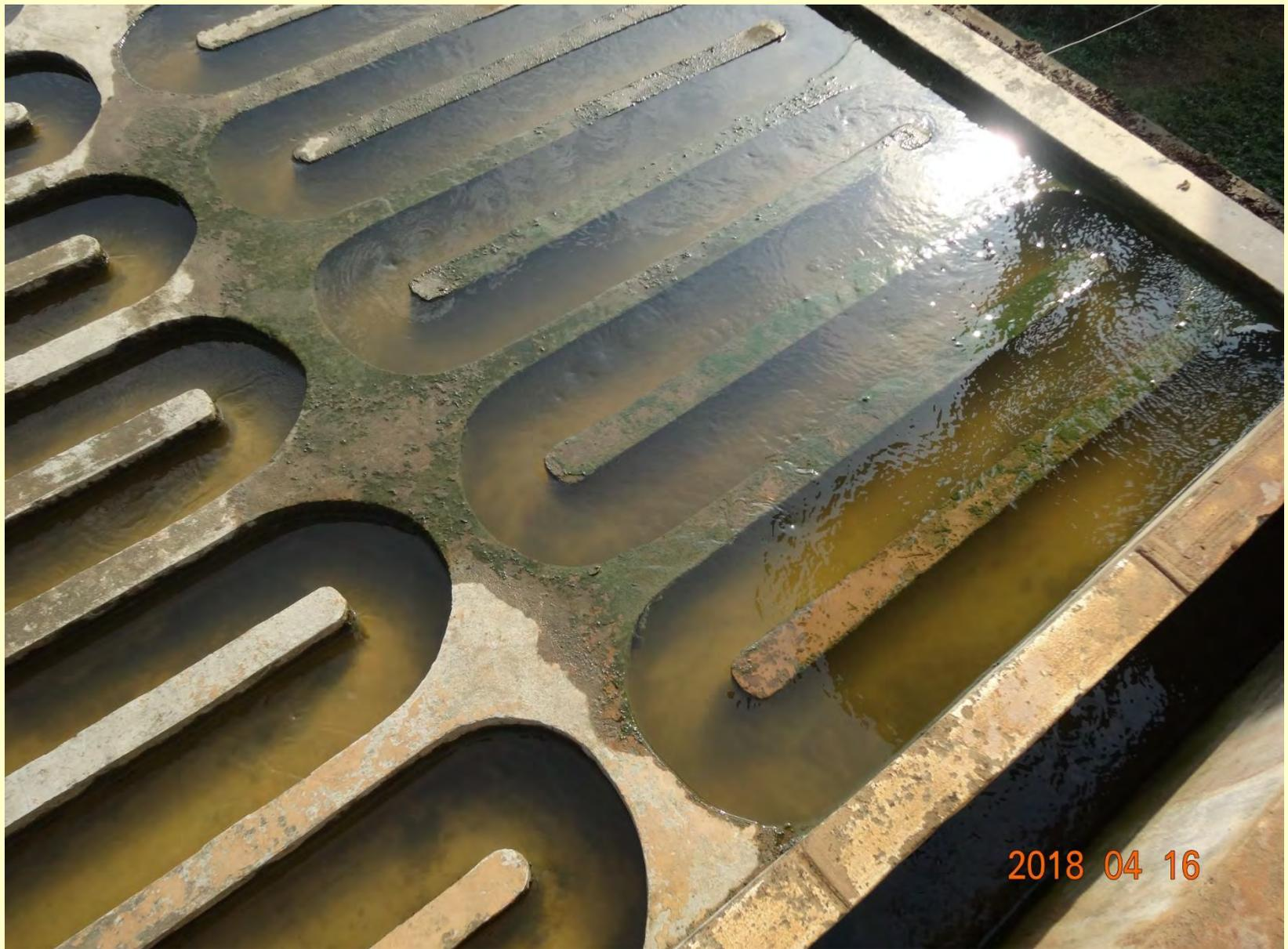
Baffling type flocculation basin with no flow, overflow, and algae attachment 24
