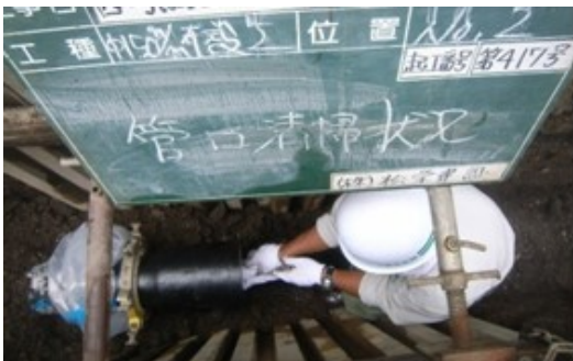
Picture 2: Cleaning inside pipe
